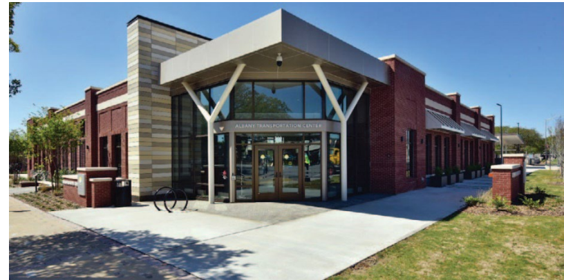
On March 27, 2023, Albany Transit System opened the downtown multimodal transit facility at 300 West Oglethorpe Blvd.
